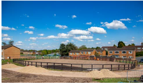
"SUDs" installation Mansfield
