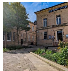
The Court House Rain Garden, Mansfield
